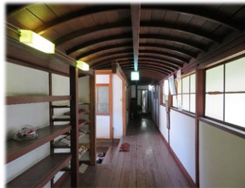
廊下舟底天井
