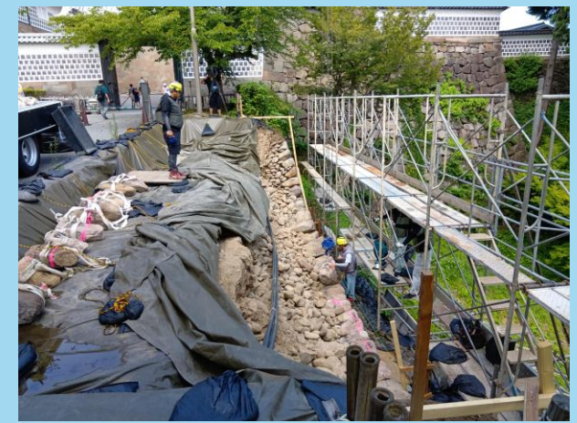
R8.8 積み直し工事
